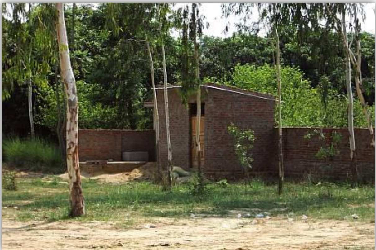
(Toilets and Storeroom)
