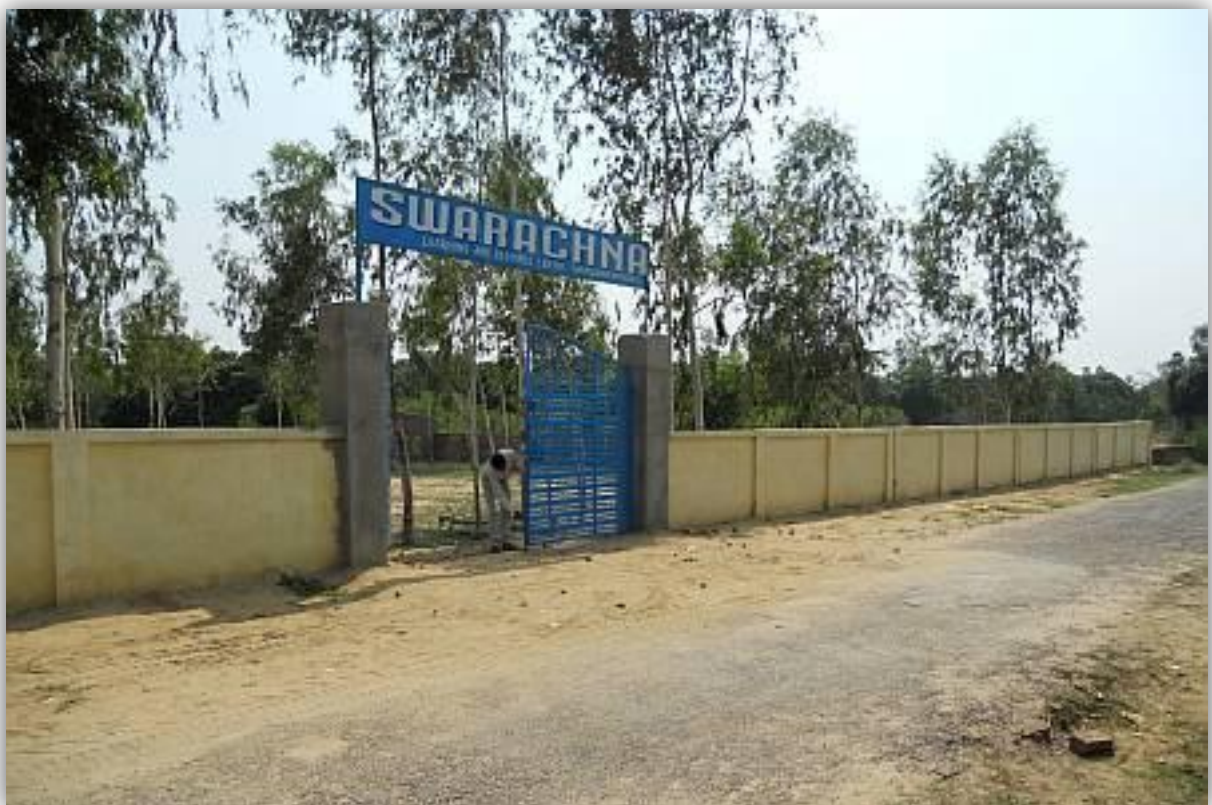
(Boundary Wall and Gate)
